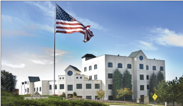
AutomationDirect's corporate headquarters near Atlanta, Georgia
